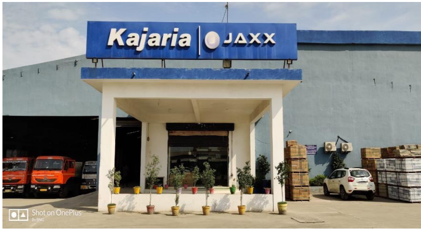
Kajaria Vitrified, Gujarat (formerly known as Jaxx Vatrified Pvt Ltd)
